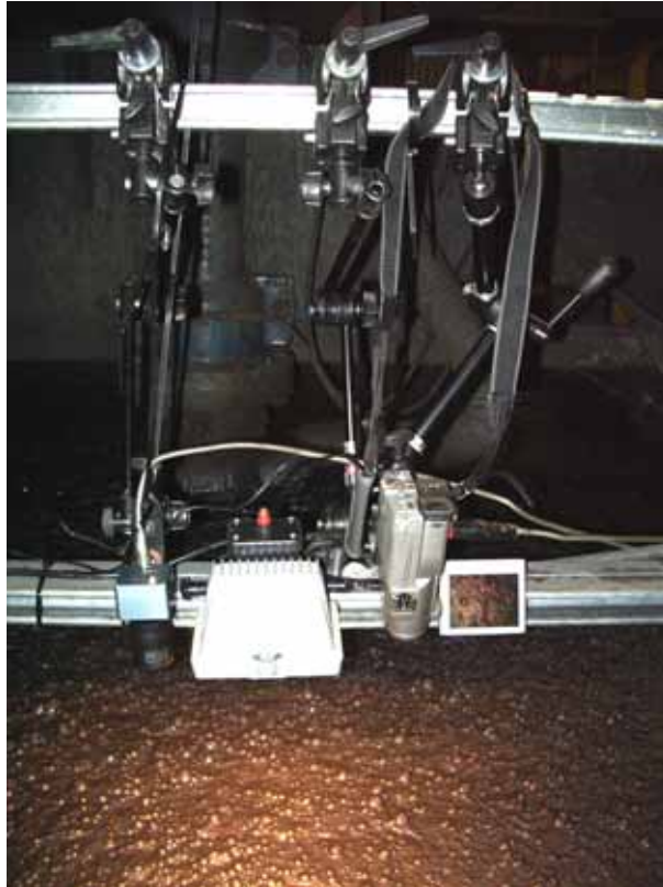
Figure 3.45: SmartFroth camera and lighting system installed on rougher 3 of the molybdenum circuit.
