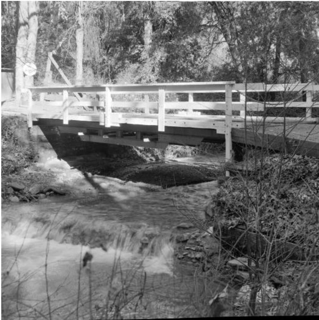
Figure E.3: Bridge.
